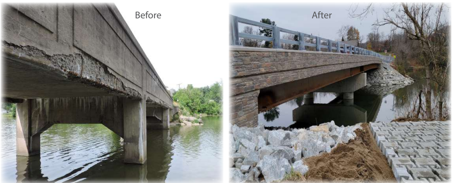
Chartiers 12 (Cannonsburg Lake) Bridge Rehabilitation; Image Courtesy of Washington County
