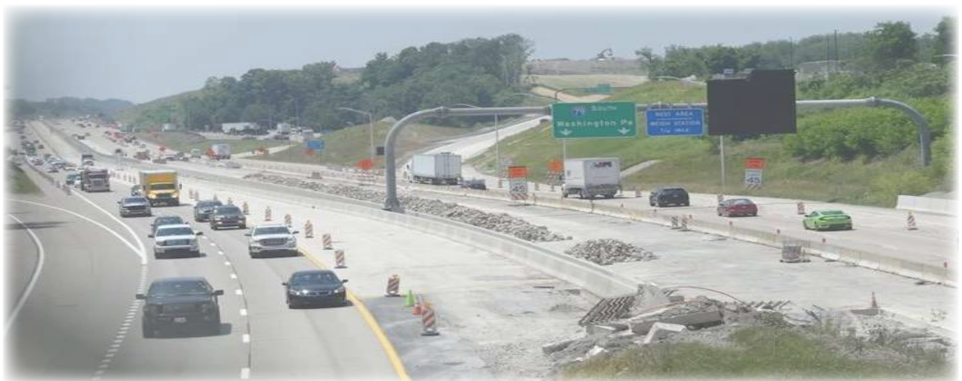
Southern Beltway Construction, Source : Observer Reporter
