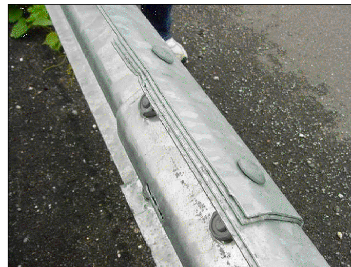
TYPICAL NESTED PANEL MID-SPAN SPLICE
